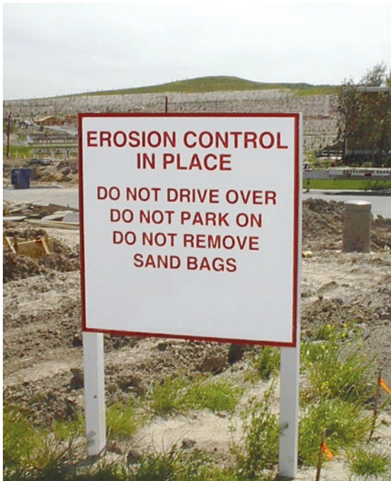
Figure 4. Use signage to help educate construction staff.
